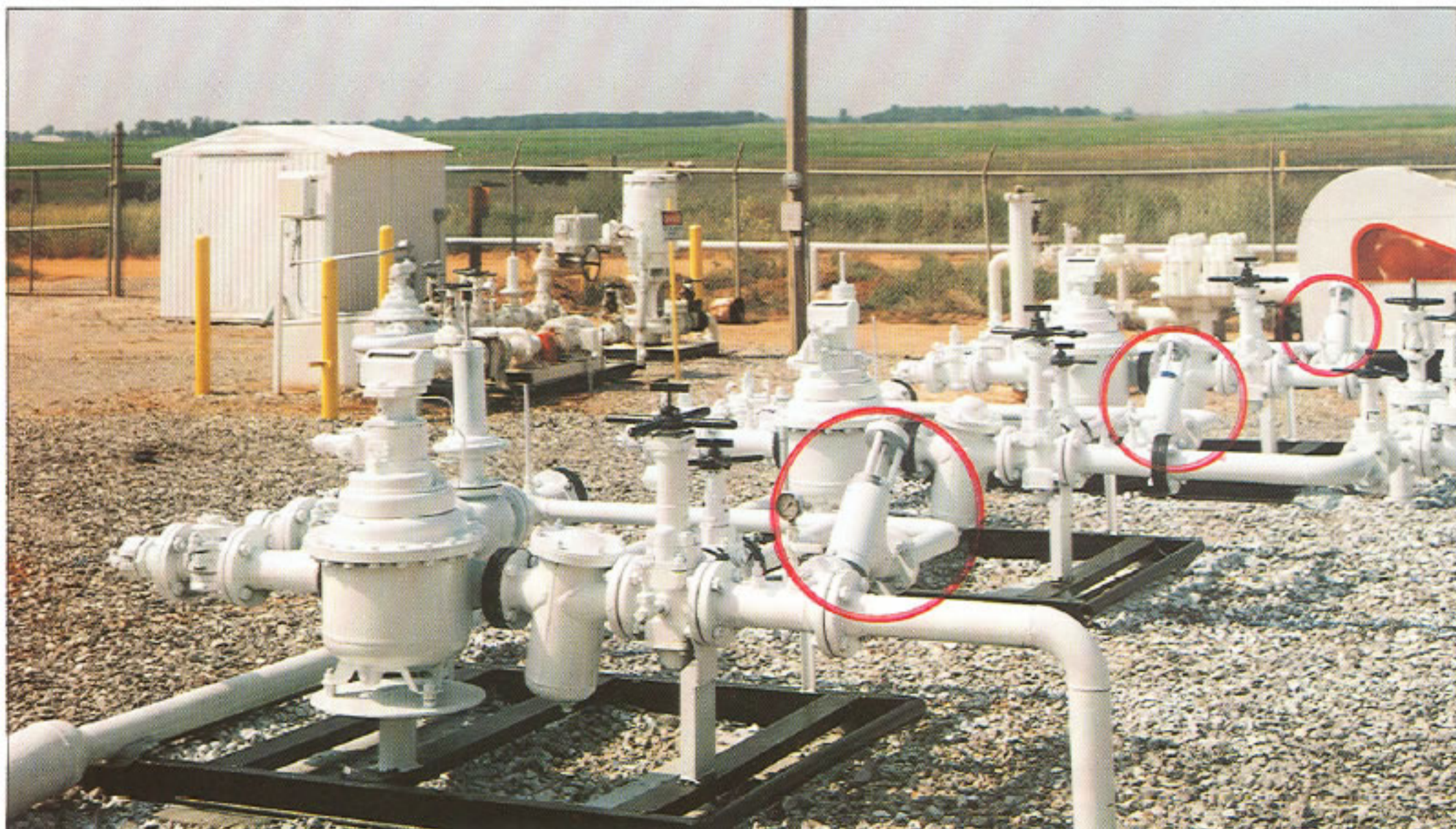
In station applications, the rupture pin valves offer protection against accidental valve closings as well as those occurring due to control valve failures.
